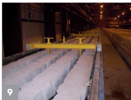
Demoulding of the hardened concrete ties
